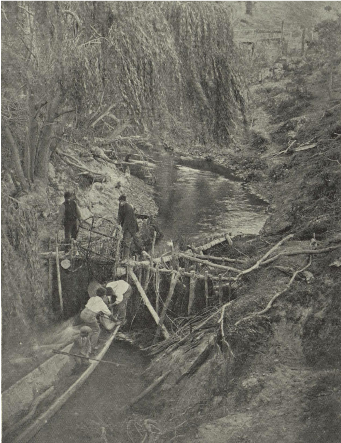
Figure 12: Small pa-tuna V type weir at Ngutuwera, Moumahaki River (Source Downes 1918 plate XIII)
