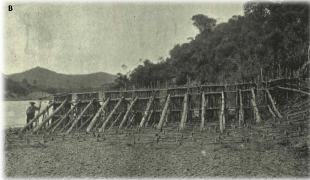
Figure 9: Utu piharau (lamprey weir) at Parikino, Whanganui River during low water flows A) looking down stream and B) looking upstream (Source Downes 1918, plate XXVII, facing p. 312).
